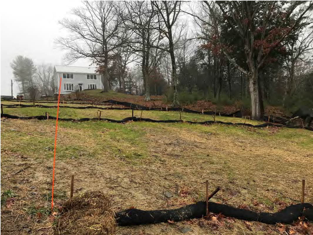
Fig 1: Slope above the cable house at the Eversource property/west side of the bay. Viewing northwest. (12-11-20)
