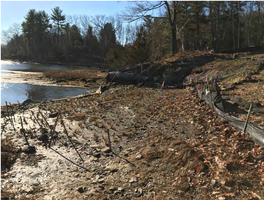
Fig 4: Toe of the slope and salt marsh restoration at the Eversource property/west side of the bay. Viewing south. (12-15-20)
