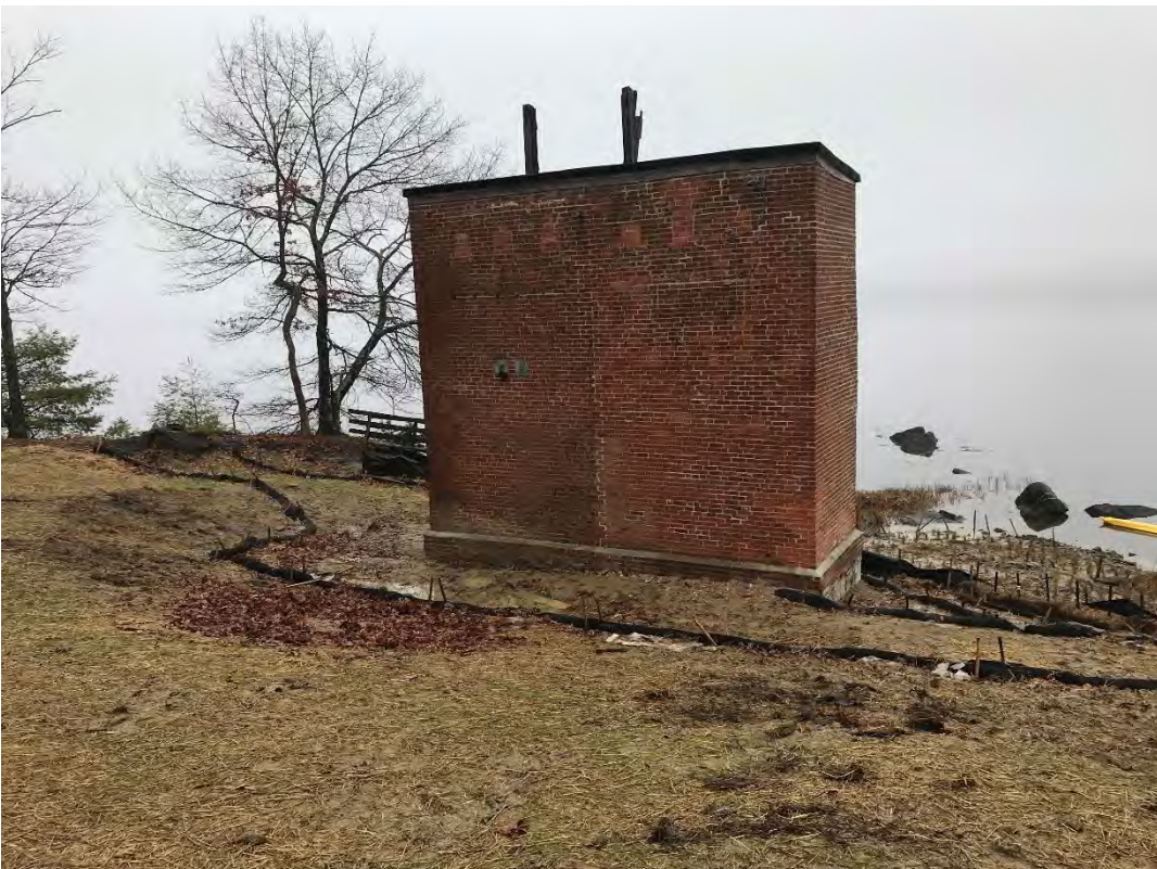
Fig 2: Slope leading down to cable house and salt marsh restoration at the Eversource property/west side of the bay. Viewing northeast. (12-13-20)
