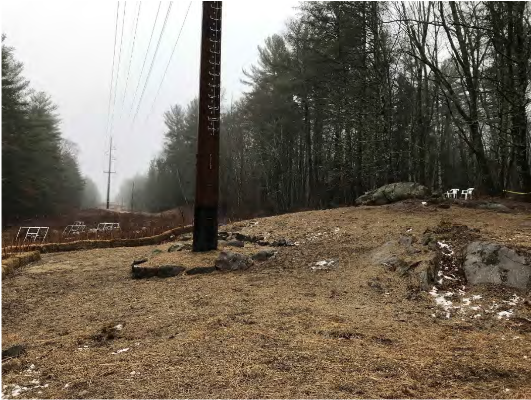
Fig 11: Str. 89 work area. Viewing southeast. (12-13-20)
